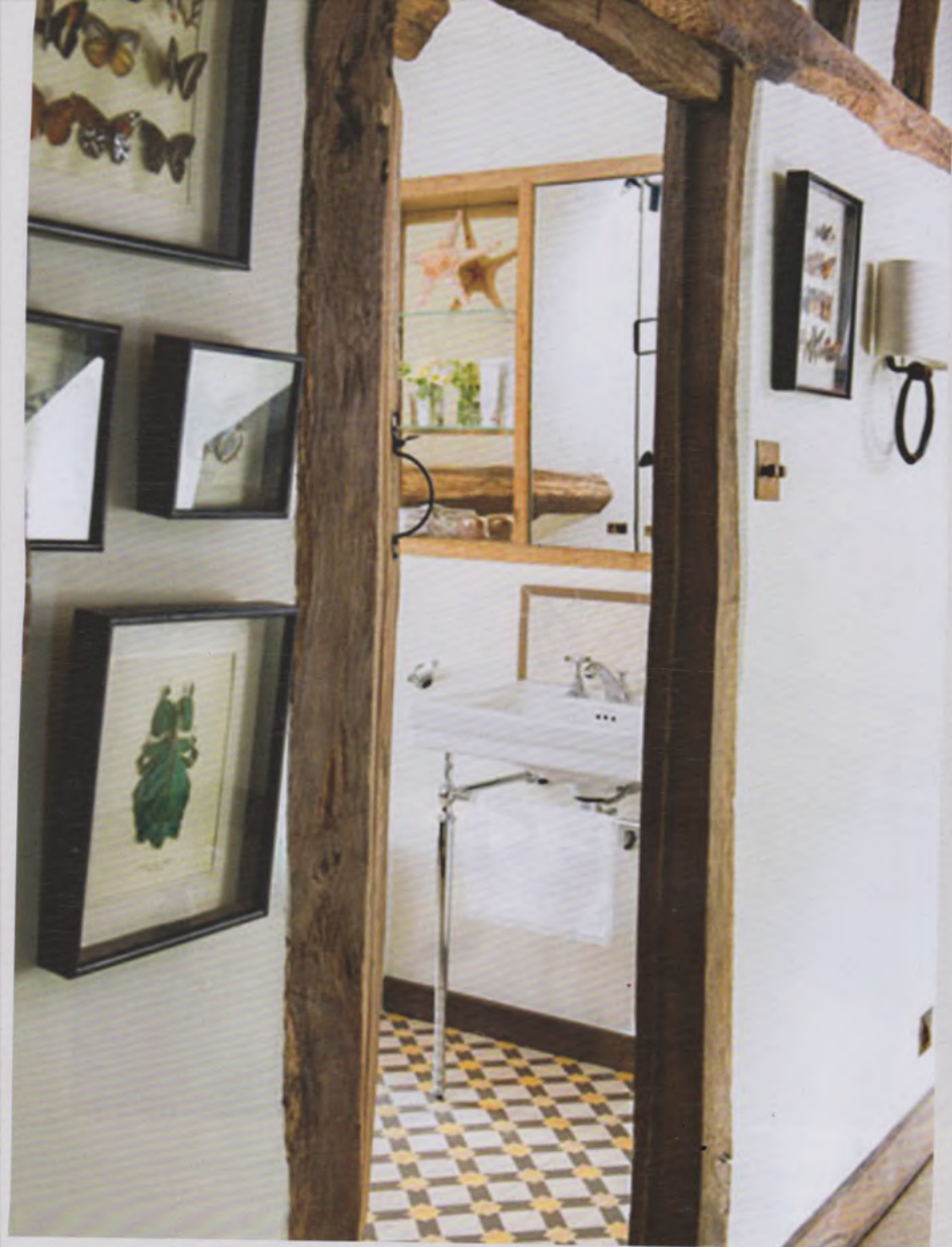
Reclaimed oak beams and joists were used to create a screen, door architraves and skirting in this 16th century cottage in Oxfordshire
